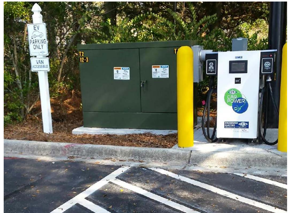
Brunswick EMC DC Fast Charge Station Calabash, NC
